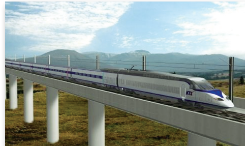
KTX 11-1 section Establishment of roadbed
