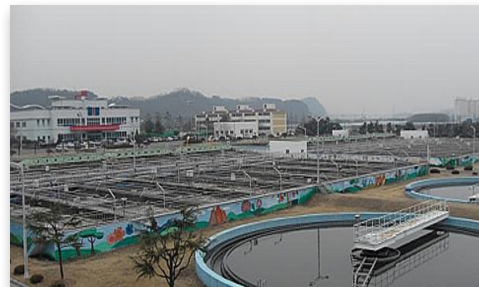
Gyeongju sewage treatment facility
